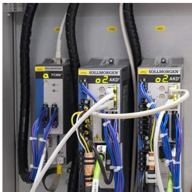
Left, KOLLMORGEN compact and high- performance PCMM controller and AKD servo amplifier. Right, the AKM servo motor capable of high acceleration.
